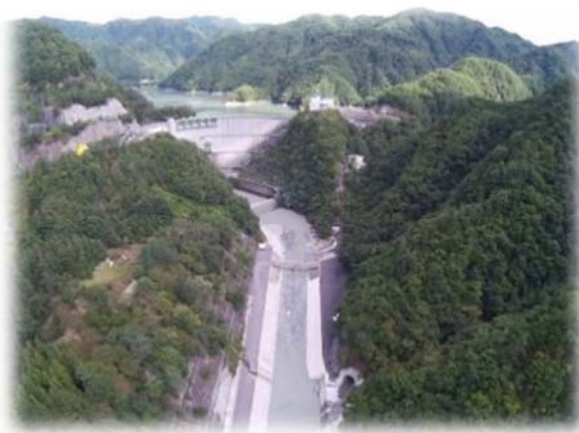
Koshiibu Dam and outlet of the sediment bypass tunnel
