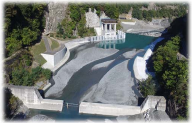
Intake of the sediment bypass tunnel and river diversion weir
